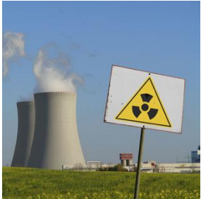
Energy: Nuclear Power Plants
